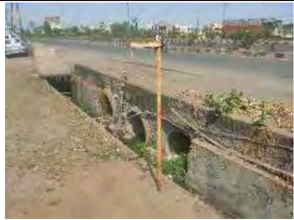
Pipe Culvert at Km 73+785
