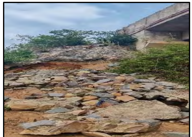
Major Bridge at Ch. 1356+285
