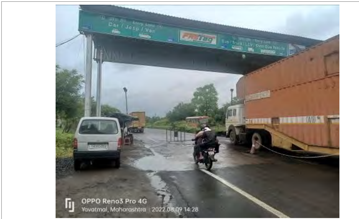
Photo 9: Electronic Toll Collection (ETC) lane
