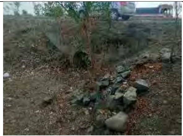
Pipe Culvert at Km 135+596
