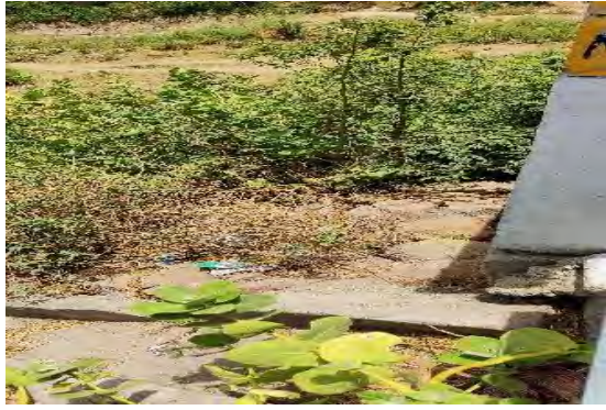
MNBR at Ch. 06+799
