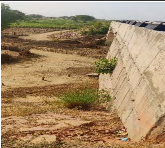
MNBR at Ch. 12+701
