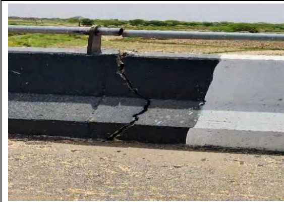
MNBR at CH.6+799
