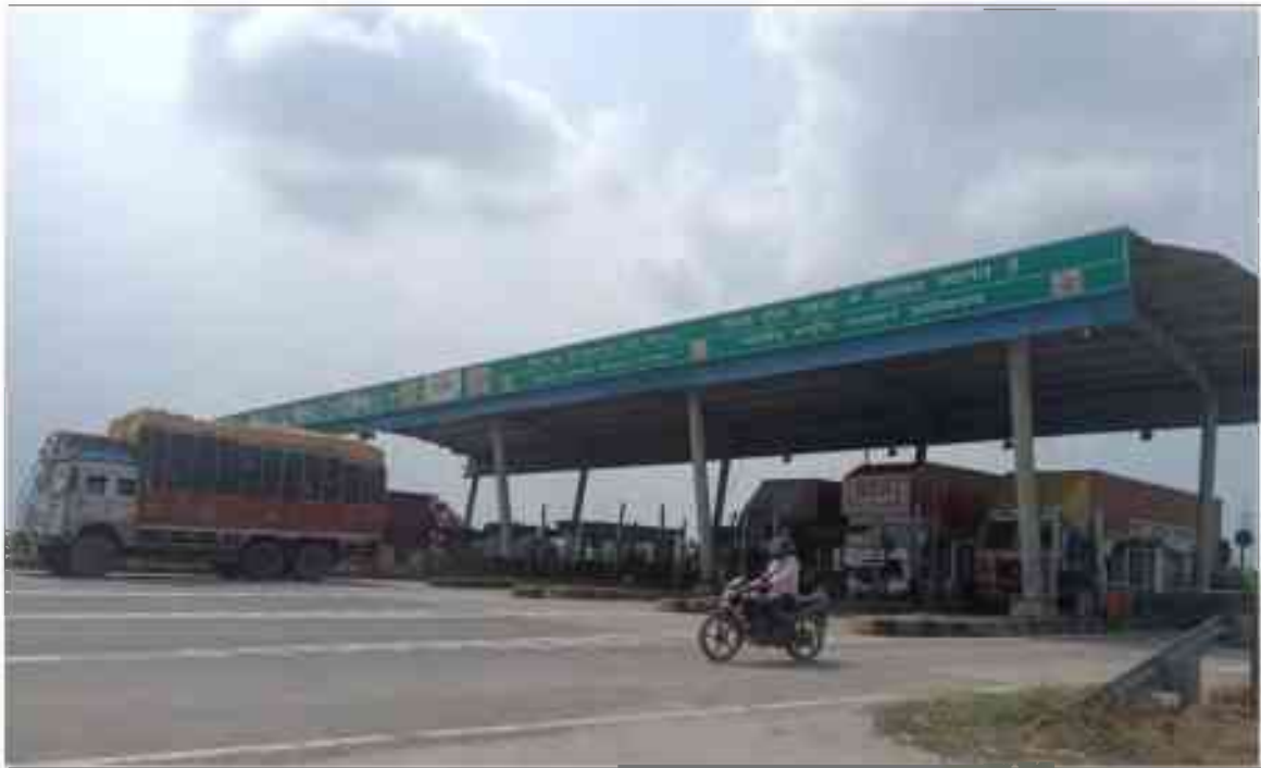
Photo 8: Raibha Toll plaza
