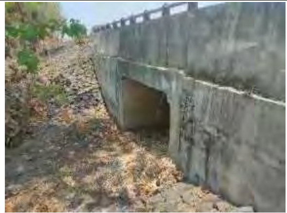
Box Culvert at Km 161+580
