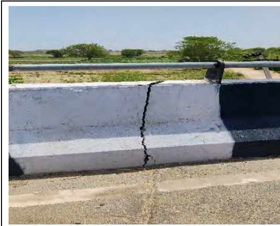
MNBR at CH.1+838
