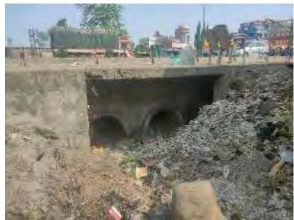
Pipe Culvert at Km 63+168
