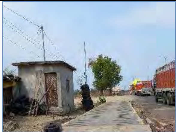
Weigh bridge, LHS @ 92+500
