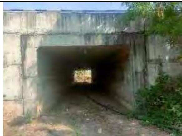
Box Culvert at Km 66+244
