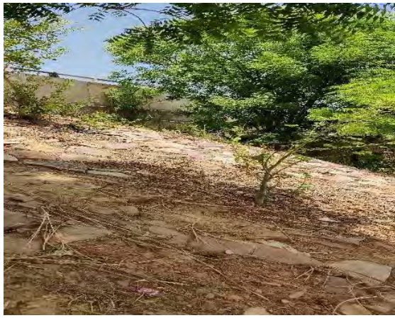
MNBR at Ch. 03+640
