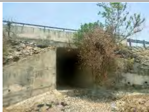
Box Culvert at Km 95+914
