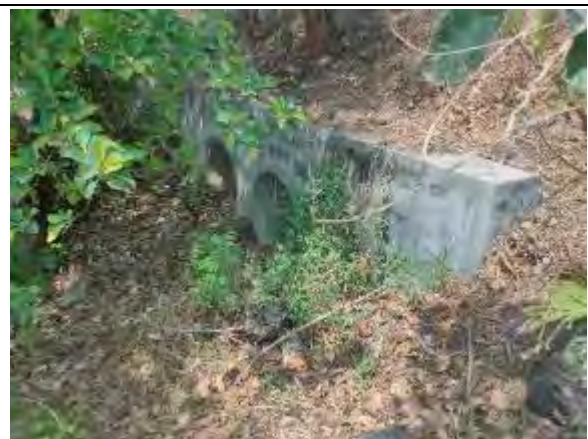
Pipe Culvert at Km 116+901
