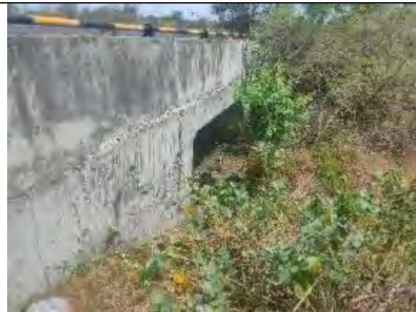
Box Culvert at Km 83+092
