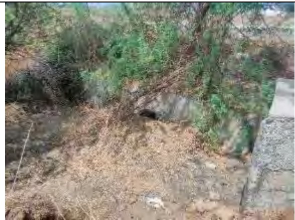
Pipe Culvert at Km 105+494
