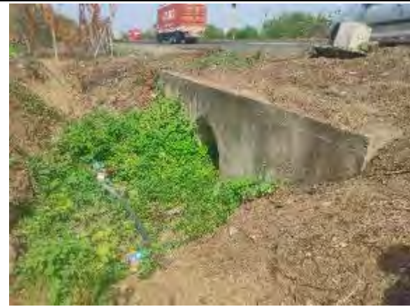
Pipe Culvert at Km 70+605
