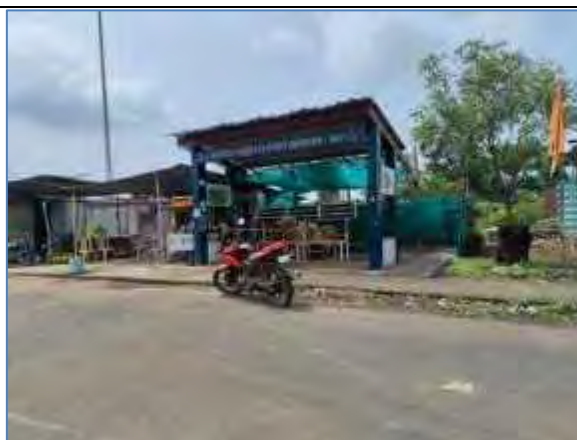
Bus shelter near km 95.526, RHS on Service Road
