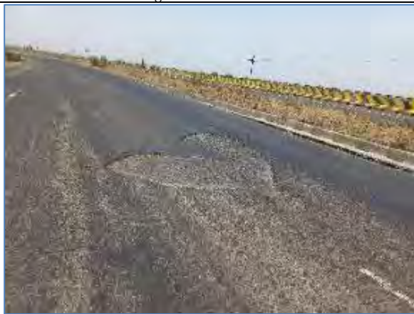
Delimitation at km 100.050-LHS
