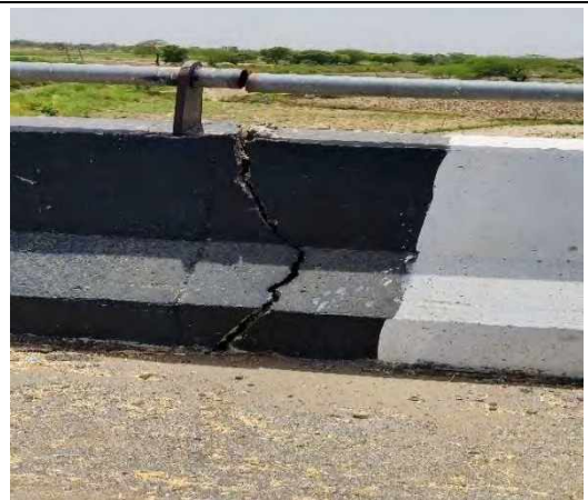
MNBR at CH.6+799
