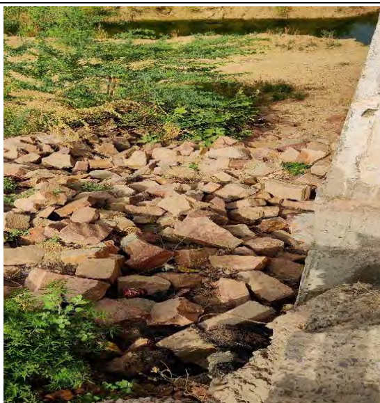
MNBR at CH. 31+547
