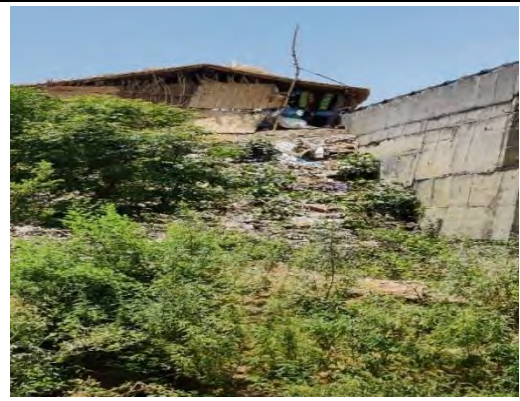
MNBR at Ch. 03+142
