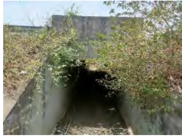
Box Culvert at Km 42+387
