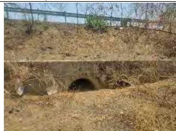
Pipe Culvert at Km 111+349
