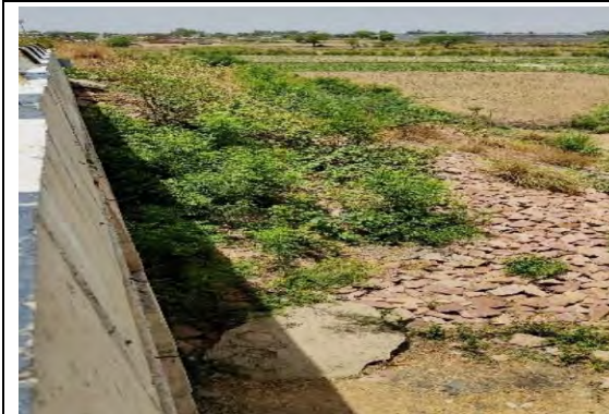
MNBR at Ch. 06+799
