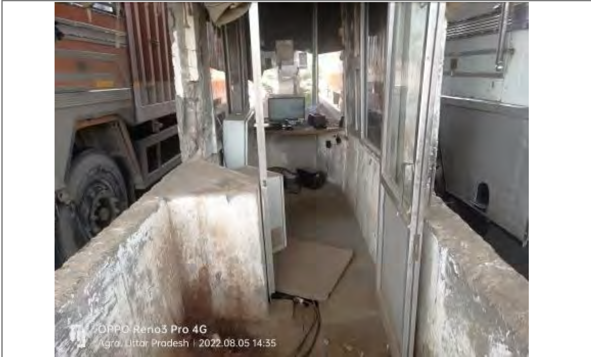
Photo 9: Inside view of toll booth
