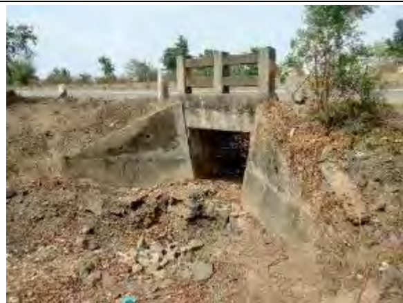
Slab Culvert at Km 57+155
