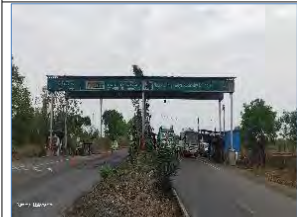
Toll Plaza at km 150+400
