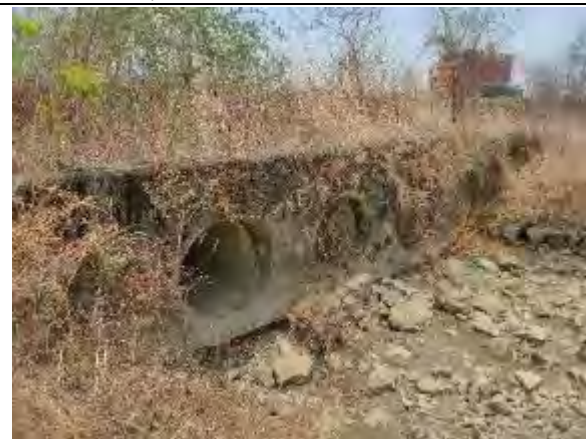
Pipe Culvert at Km 40+262
