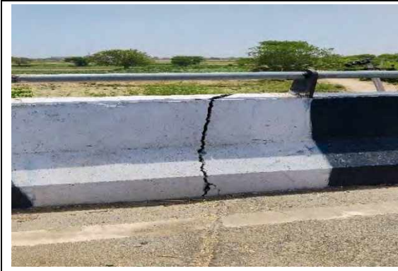
MNBR at CH.1+838
