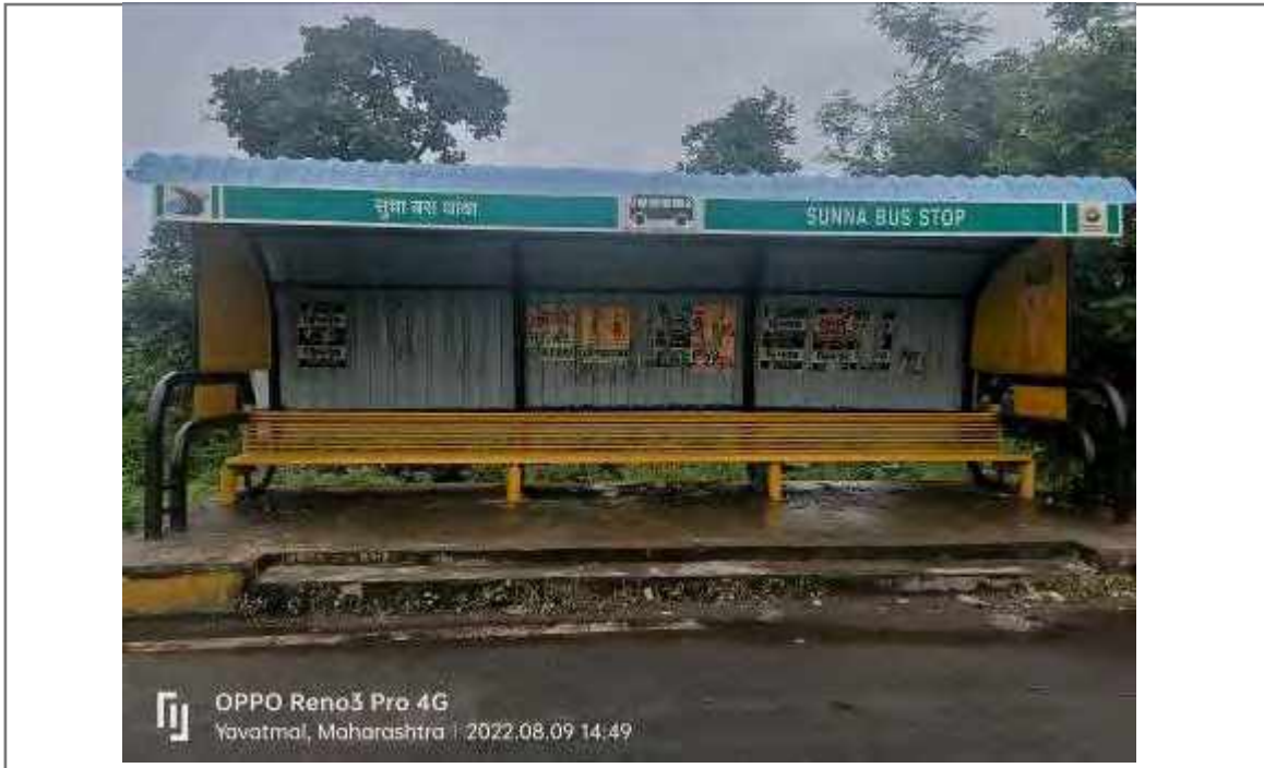
Photo 10: Bus stop along National highway
