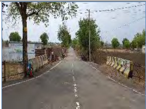
Minor Junction at km 108.700 LHS
