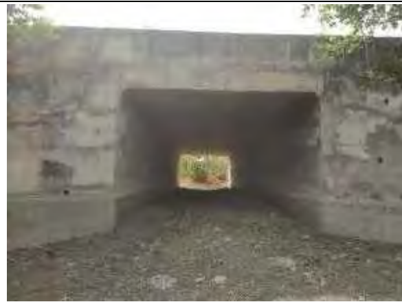
Box Culvert at Km 130+662
