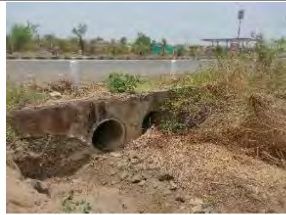
Pipe Culvert at Km 38+483
