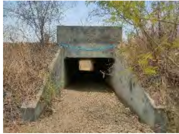
Box Culvert at Km 41+016
