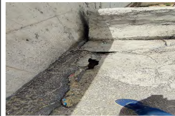
ROB at CH 8+954 Settlement pass
