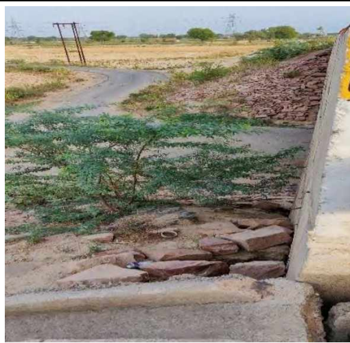
MNBR at Ch. 15+661
