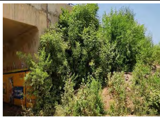
MNBR at Ch. 08+183
