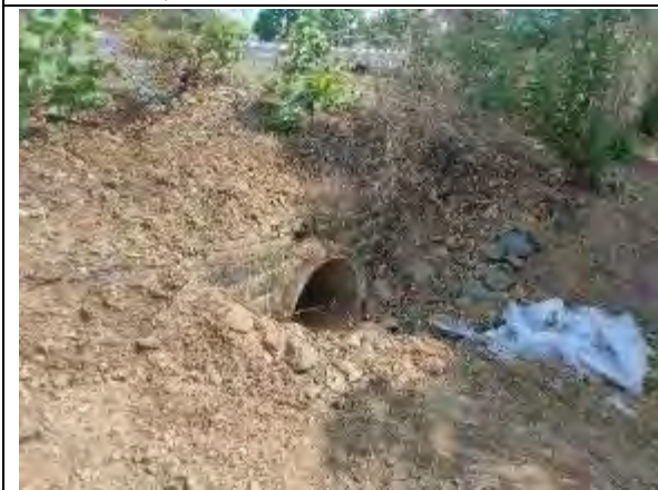
Pipe Culvert at Km 127+180
