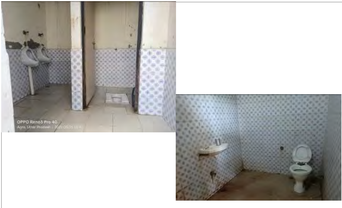
Photo 6: Toilet facilities at the toll plaza
