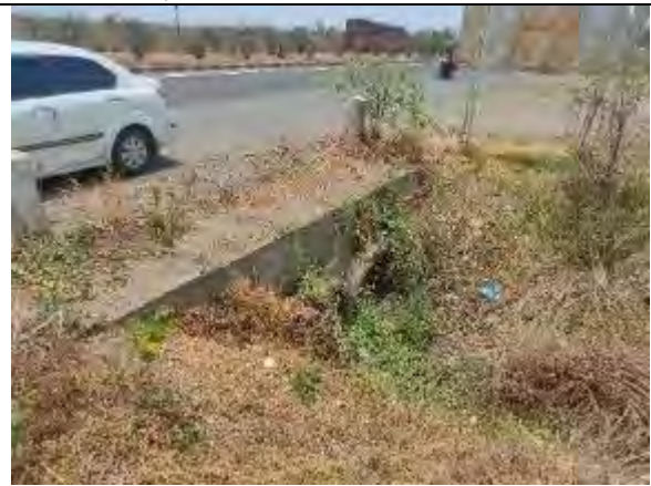
Pipe Culvert at Km 43+166
