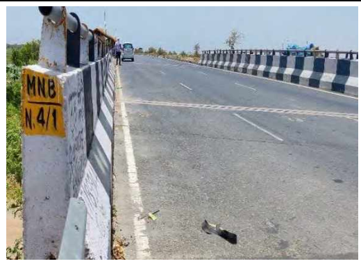
MNBR at CH. 3+142
