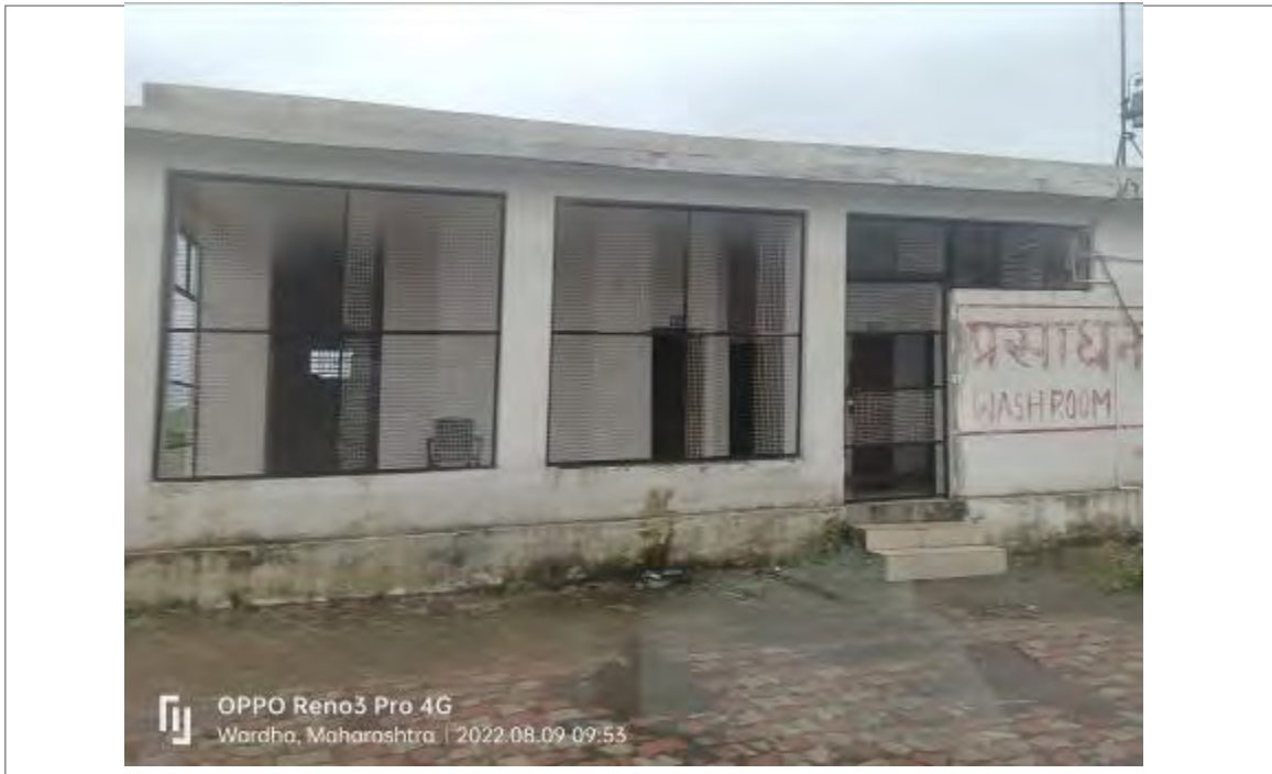
Photo 7: Washroom facility on the toll plaza
