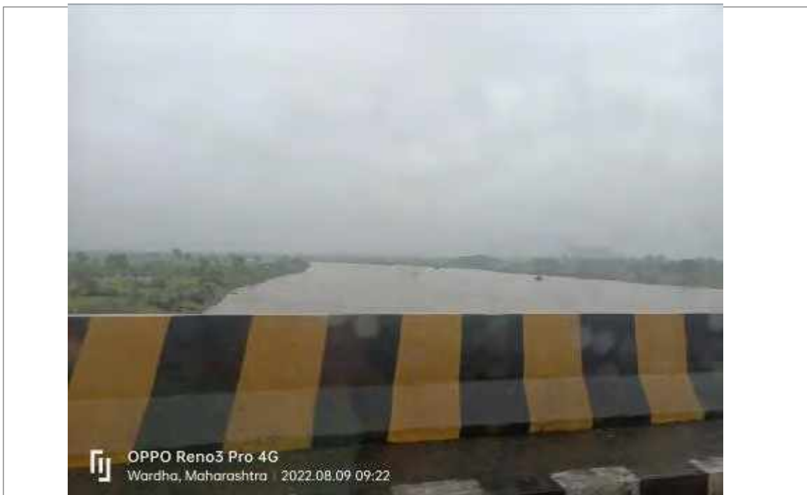
Photo 2: Bridge over the river in project area
