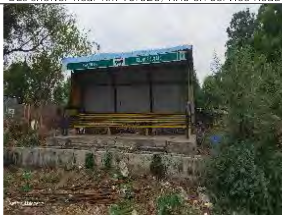
Bus shelter near km 153.090 on Service Road, LHS
