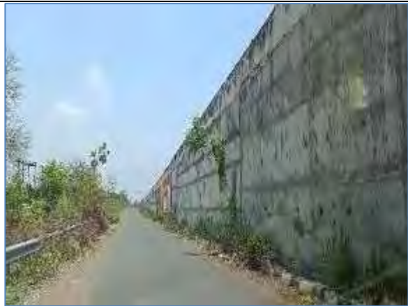
Service Road @ km 66.700 to km 67.350-LHS_5.5m wide
