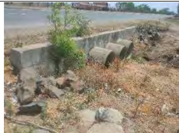
Pipe Culvert at Km 90+720
