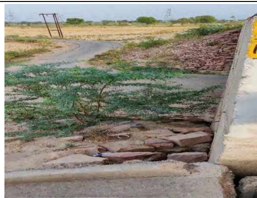
MNBR at Ch. 15+661
