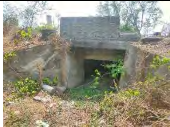
Slab Culvert at Km 51+180
