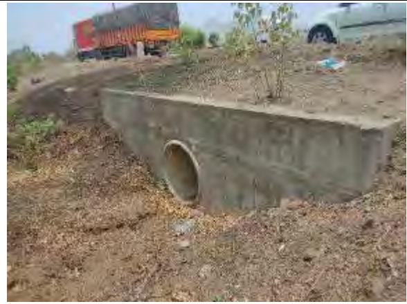
Pipe Culvert at Km 39+249
