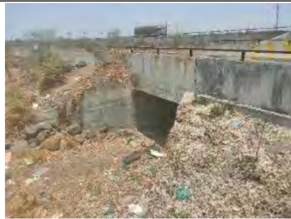
Box Culvert at Km 100+121
