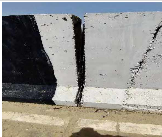
ROB at CH 8+954
