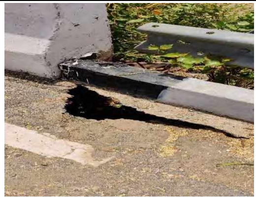
MNBR at CH 6+799
