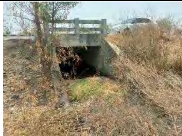
Slab Culvert at Km 46+847
