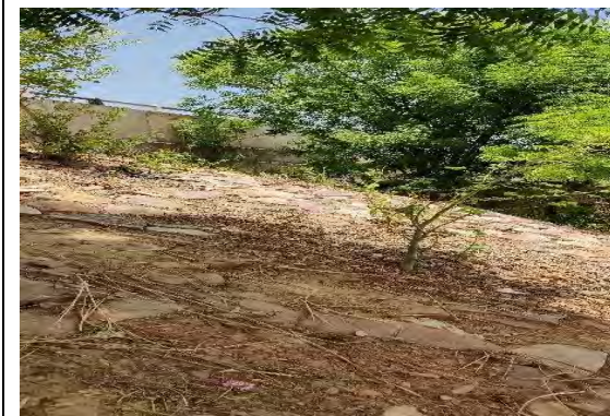
MNBR at Ch. 03+640
