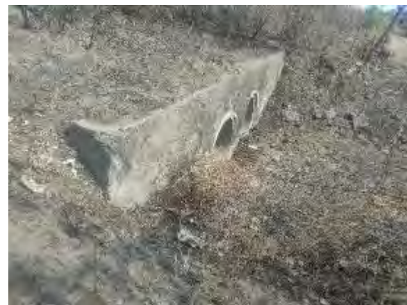
Pipe Culvert at Km 61+789
