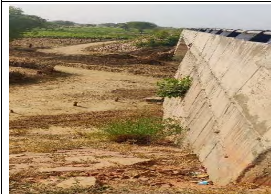
MNBR at Ch. 12+701
