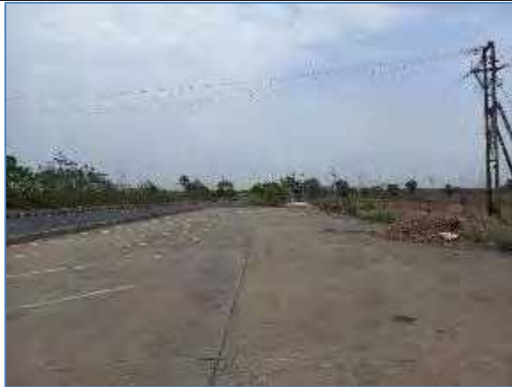
Truck Lay bye on LHS km 68.240
