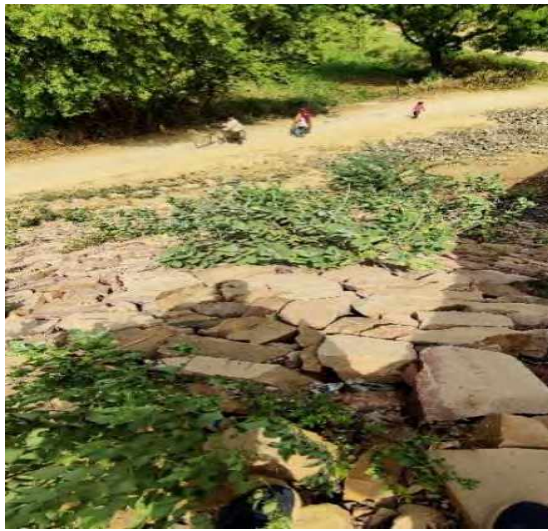
MNBR at CH. 17+661
