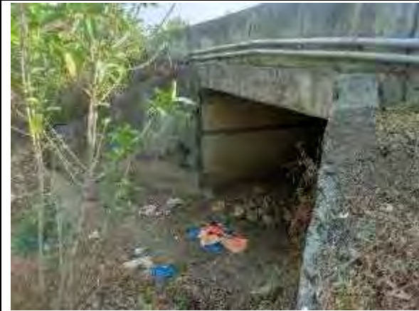
Box Culvert at Km 147+032
