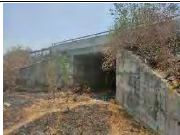
Box Culvert at Km 93+985
