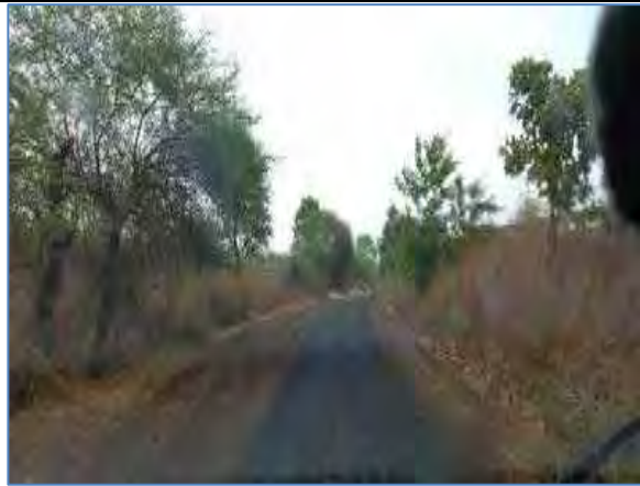
Service Road @ km 128.800 to km 129.150 - LHS_5.80m wide
