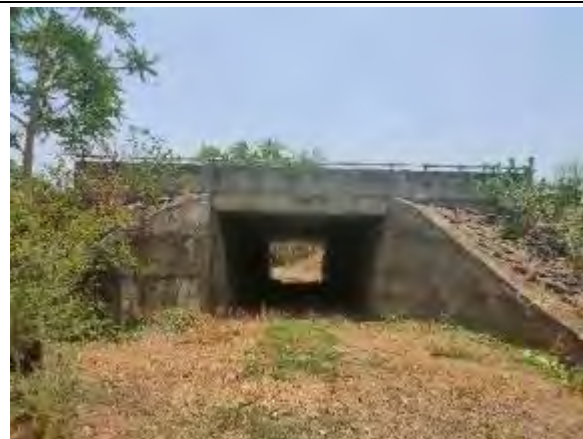
Slab Culvert at Km 164+145
