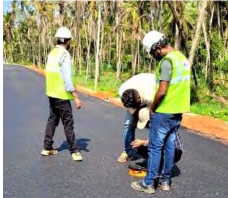
Asphalt Density Guage Tester at Perambra Bypass
