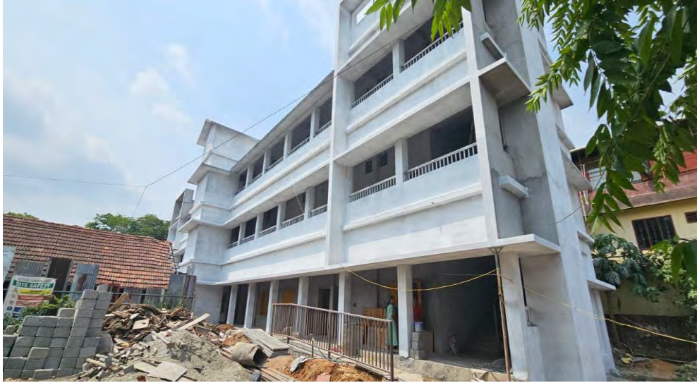
Fig 4.2 Academic block in progress
