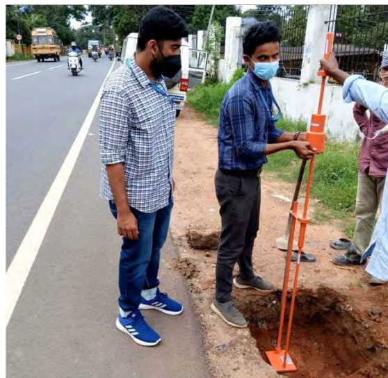
DCPT Test at Vazhimukku- Kaliyikkavila Road
