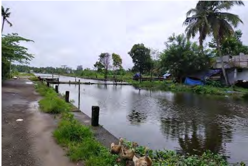
Fig 21.1 Phase I canal cleaning
