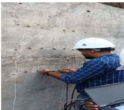
Ultrasonic Pulse Velocity (UPV) Test at Moolethara Canal, Palakkad
