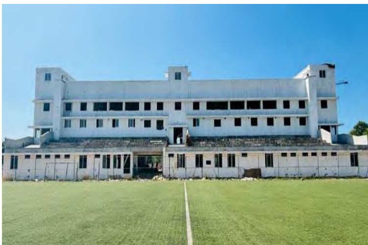
Fig 8.2 Pavilion gallery under construction
