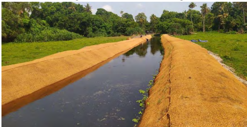
Fig 21.2 Phase II canal cleaning
