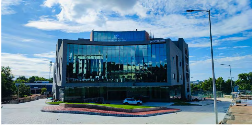
Fig 19.2 Technology Innovation Zone Building 1 at Kochi Innovation Zone
