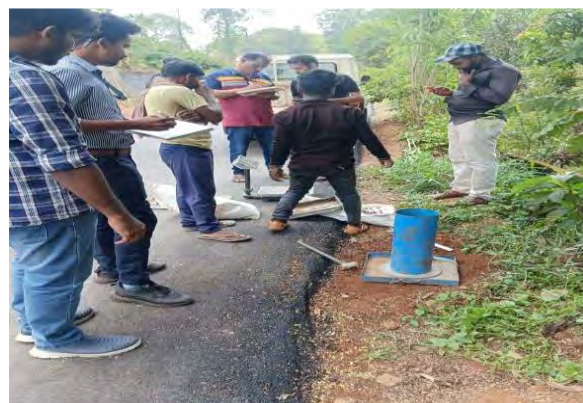
Field Dry Density (FDD) Test in shoulder
